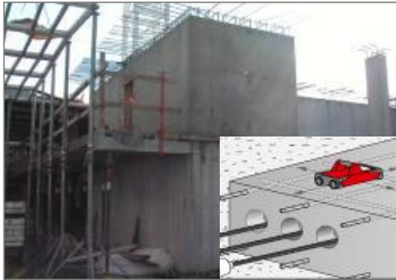
Drilling/coring / Assessing in concrete structures
