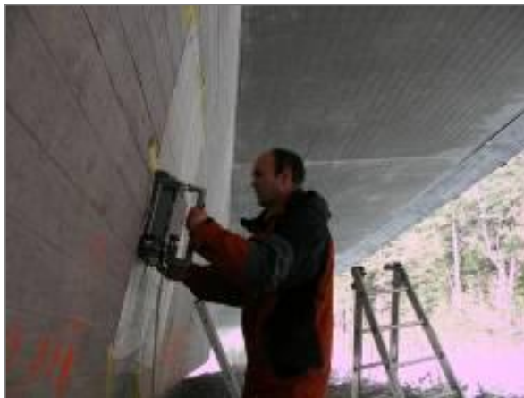
Non-destructive inspection of bridges e.g. location of tendons
